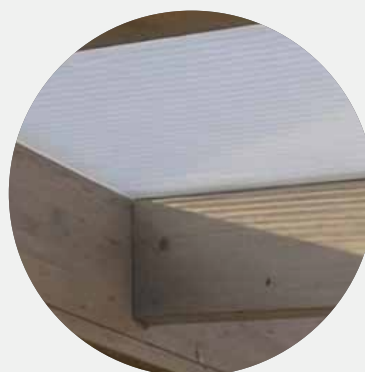
Lysinslipp i taket
